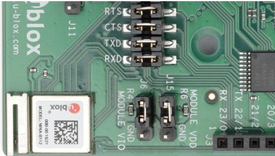
Figure 9: Placement of R4 and R6 (10 \Omega resistors)
