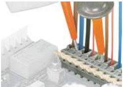
Testing with test probes.
