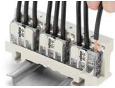
Removing a conductor.
